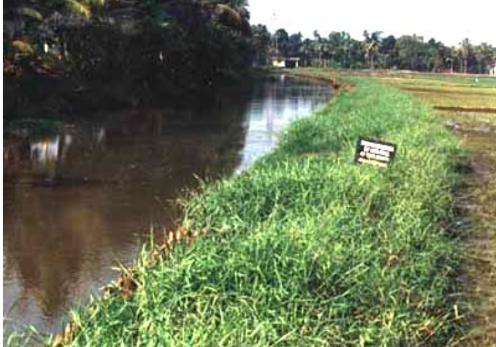
Fig.6. Fully protected mud wall due to established vegetation
