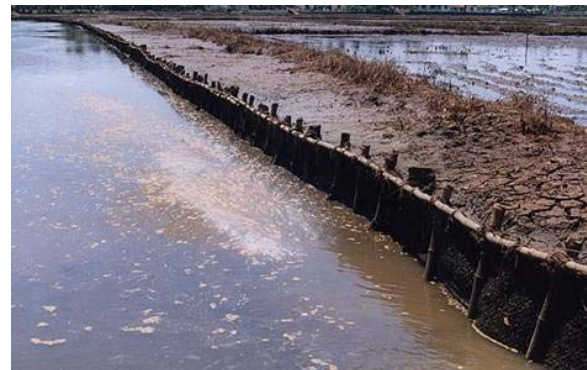
Fig. 2. Application of coir geotextile using bamboo poles
