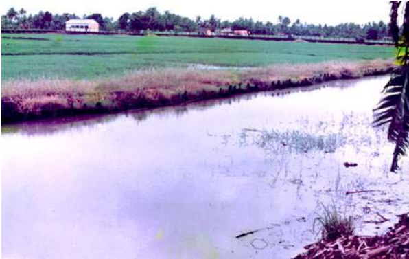
Fig. 5. Reinforced mud wall with grown vegetation after 8 years
