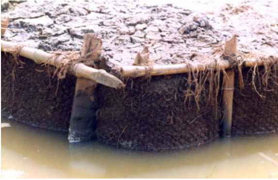
Fig.3. Close up view of applied coir geotextile on the stream bank
