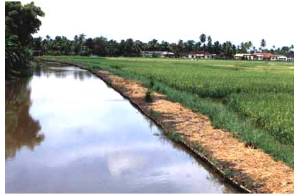
Fig. 4. Mud wall using coir geotextile at Kuttanad
