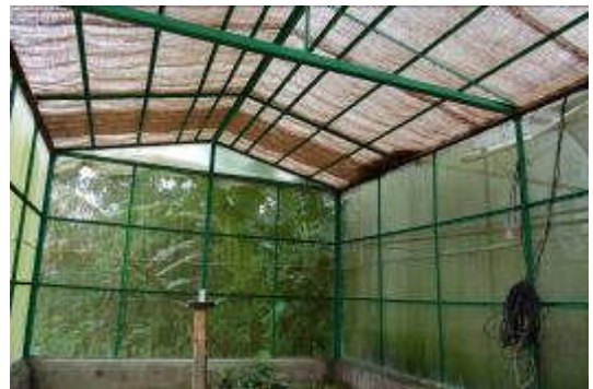
Pic 06. Polyhouse lined with 100% coir net (50% shade)
