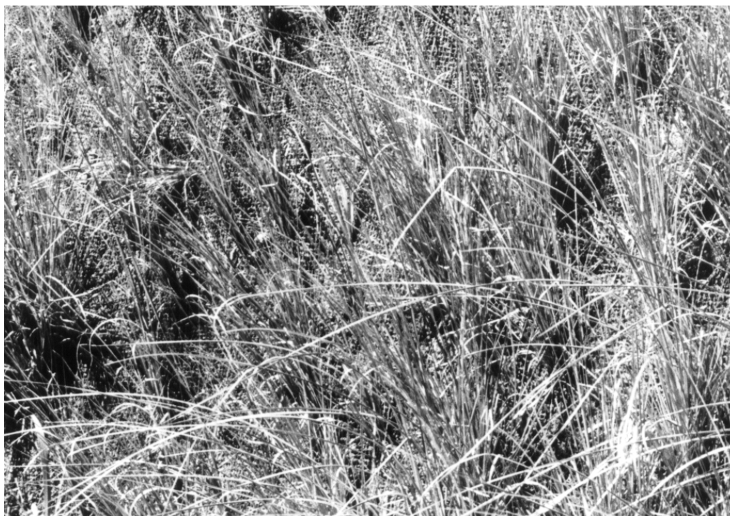
Figure 8(b). A close up view of the protected slope with the coir geotextile.
