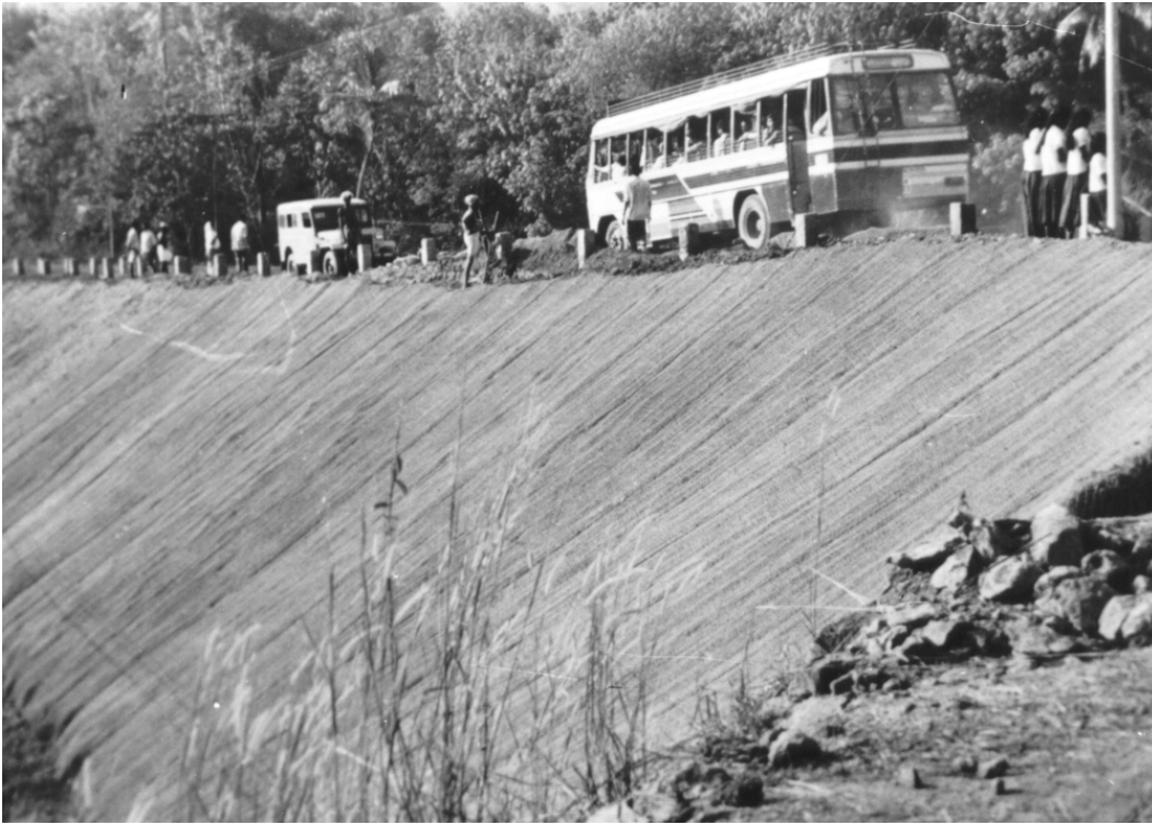
Figure 6(a). Laying of coir geotextile at the road slope at Moovattupuzha.
