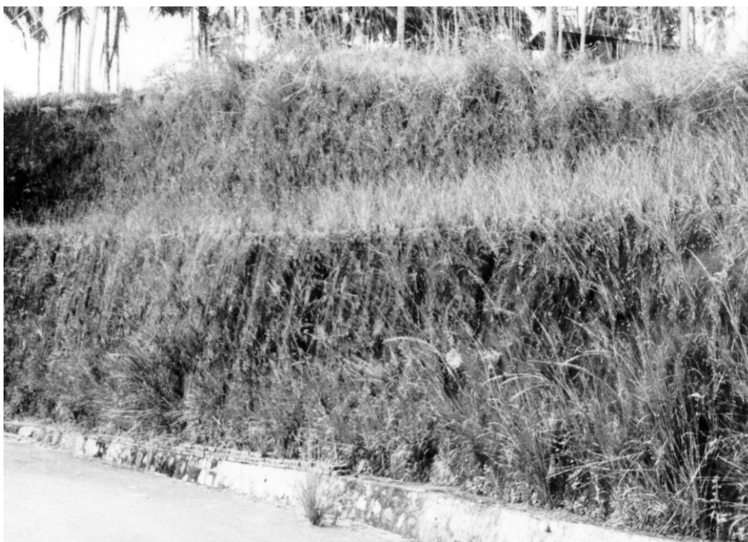
Figure 8(a). Road slope protection at Elite Gardenia, Trichur, Kerala by coir geotextile.
