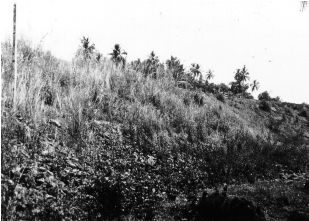
Figure 6(b). The road slope at Moovattupuzha after protection with the coir geotextile.
